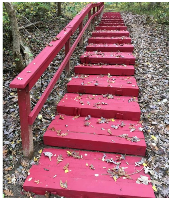
Staircase with anti-slip paint applied
